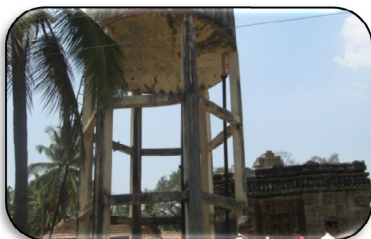
Jain Basadi, Chikmagadi, Shikaripur taluk, Shimoga district with a huge community water tank in front of the monument
